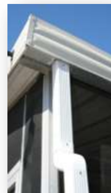
Samples of gutter transition assemblies with traditional gutters
